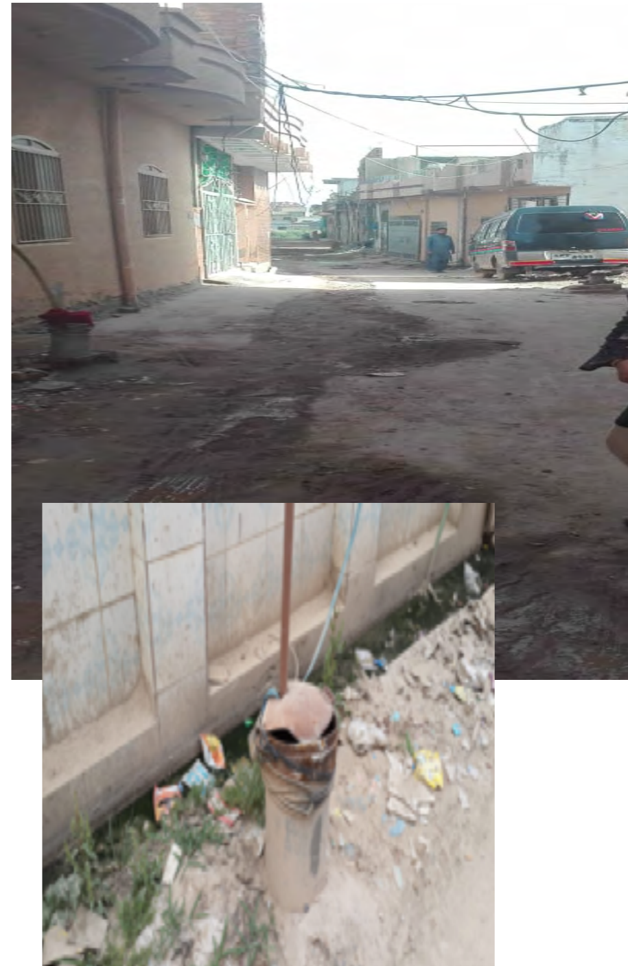
Figure 6.3. Photos of the Affected Area showing the Water, Drainage, and Sewage Systems
